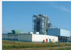
Tomakomai Power Plant
