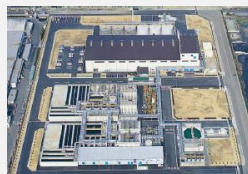
Waste liquid treatment plant
