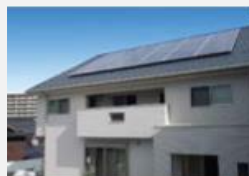
Residential solar power generation system
