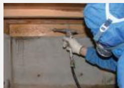
Termite control construction
