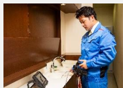
Endoscopic inspection of the inside of the water supply and drainage pipes
