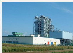
Tomakomai power plant
