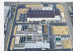
Waste liquid treatment plant
