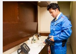
Inspection of the inside of the water supply and drainage pipes
