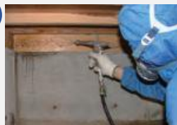
Termite control construction
