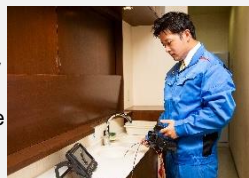
Water Pipe Inspection Using a Video Scope
