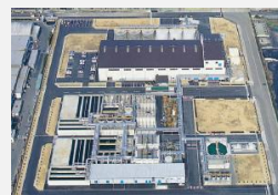
Wastewater Treatment Plant
