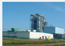
Tomakomai Power Plant
