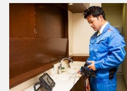
Water Pipe Inspection Using a Video Scope
