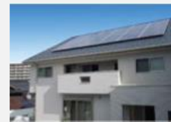
Residential Solar Power Generation System
