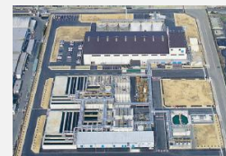
Wastewater Treatment Plant
