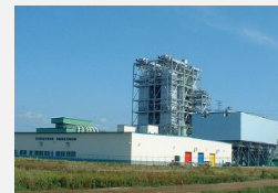
Tomakomai Power Plant
