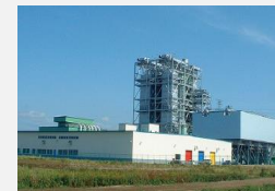
Tomakomai Power Plant
