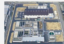
Wastewater Treatment Plant
