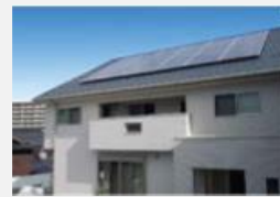
Residential Solar Power Generation System
