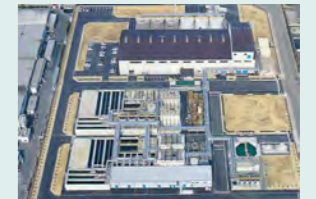
Hibiki Factory (Organic waste liquid treatment factory)
