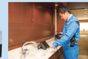
Endoscopic inspection of the inside of the water supply and drainage pipes
