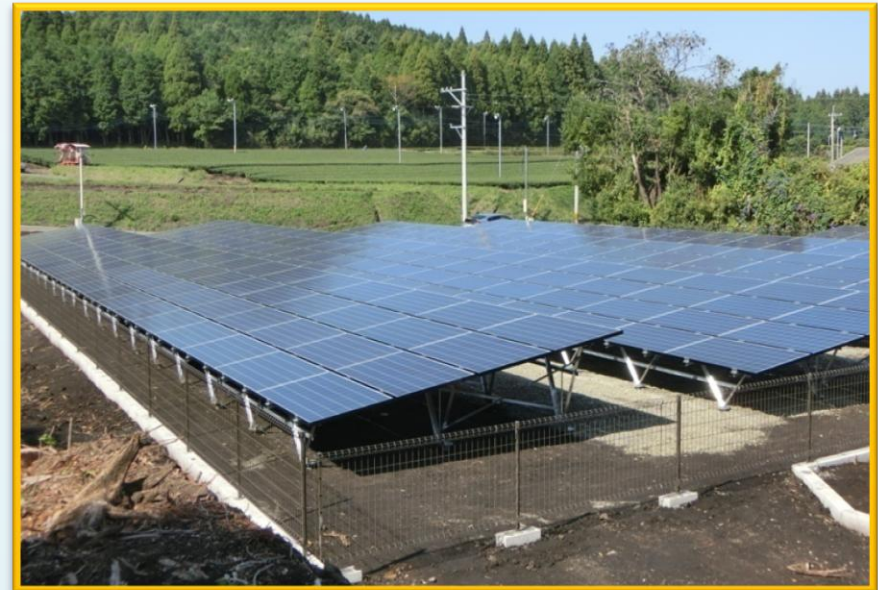
a sample of ground mounting Commercial PV system
